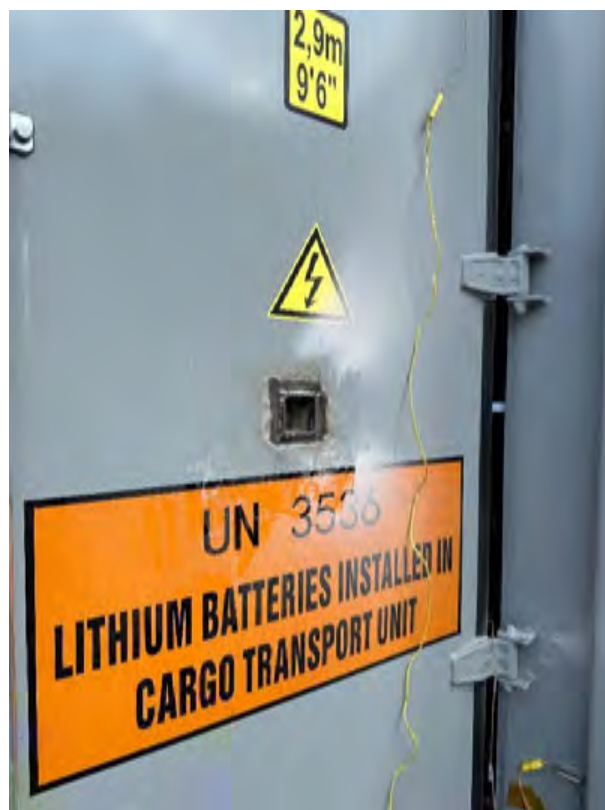
Figure 4-15 Pressure transducer well exterior
