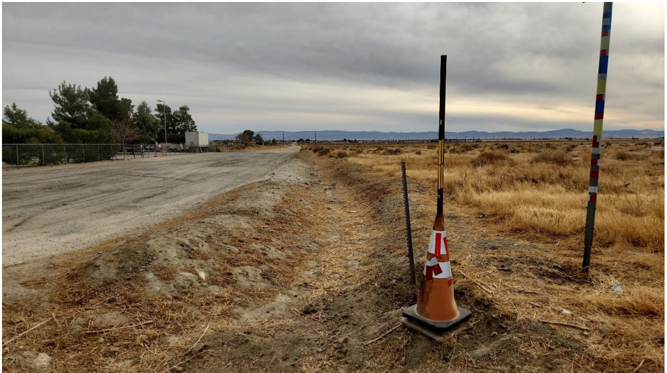
Photo Drainage 33-1. Looking south at upstream portion of Drainage 33, a roadside drainage ditch along the west side of 65 th Street W. Depicted is an artificially created berm.
