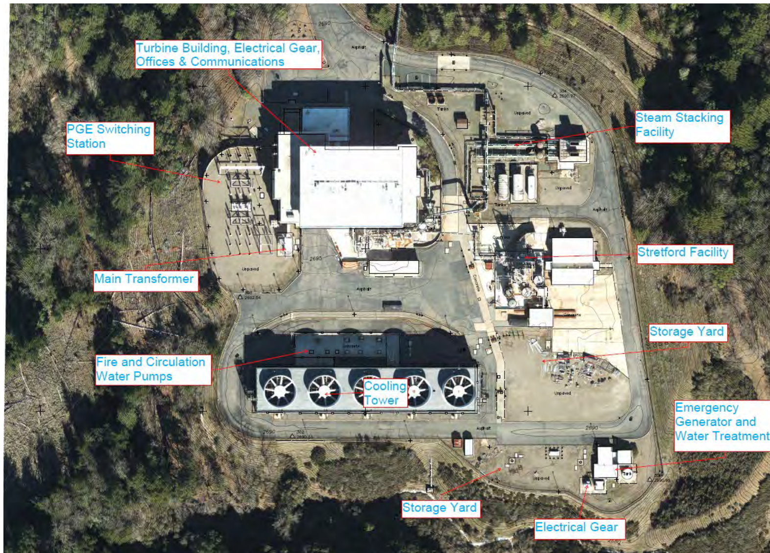
Figure 2.2-2 Existing Bottle Rock Power Plant Facilities
