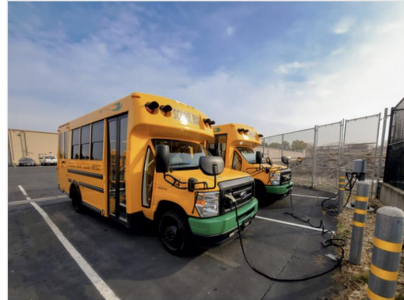
School buses charging at the Pittsburg Unified School District bus depot. Photo provided by Pittsburg USD.
