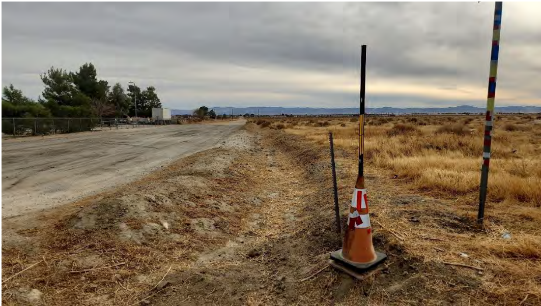
Photo 101. Looking south at upstream portion of Drainage 33, a roadside drainage ditch along the west side of 65 th Street W. Depicted is an artificially created berm.
