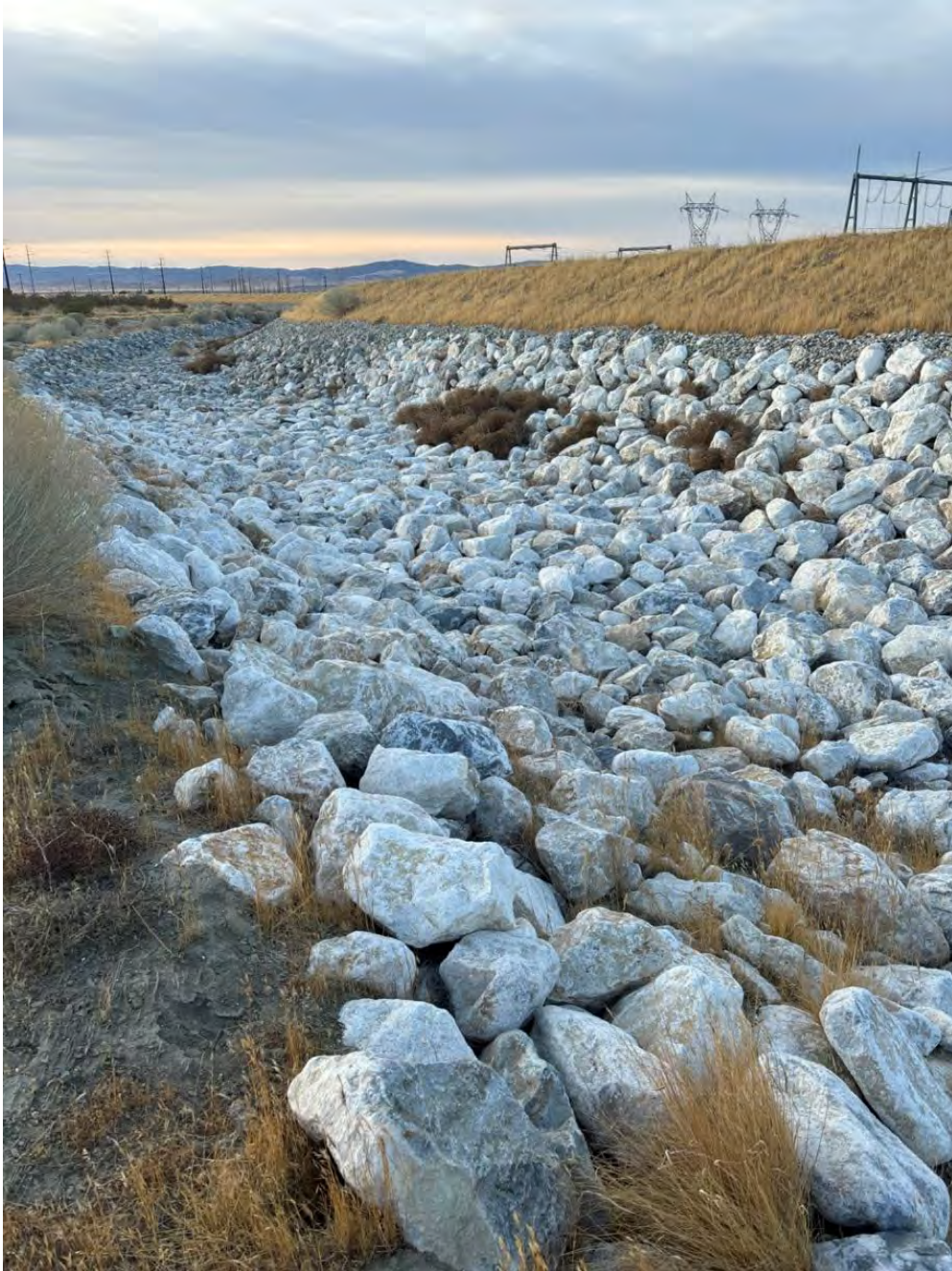
Photo 5. Looking south at Drainage 2b along the eastern side of the SCE substation. This feature is considered a flow diversion for the electrical facility.
