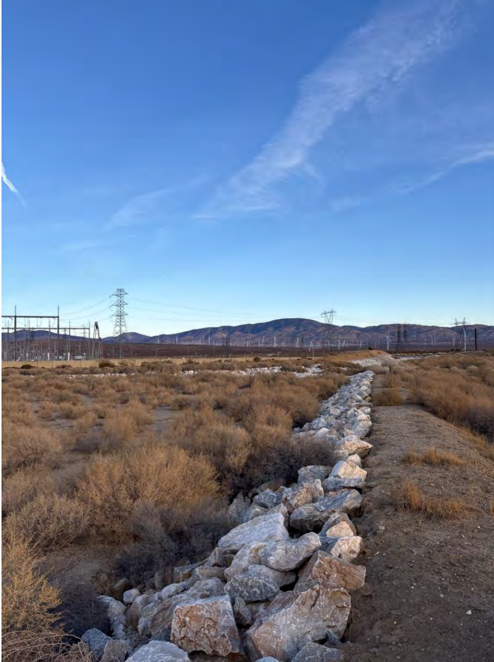
Photo 6. Looking north at Drainage 2b along the southeastern side of the SCE substation. This feature is considered a flow diversion for the electrical facility.
