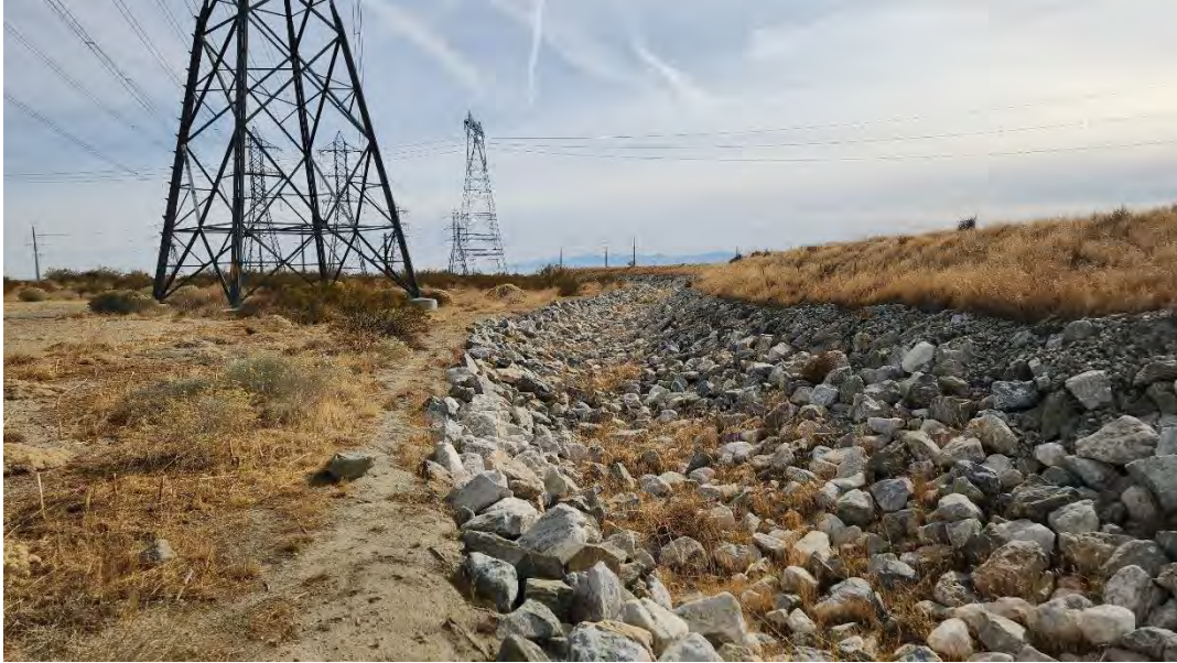
Photo 3. Looking southeast at Drainage 2a from the northeast corner of the SCE Whirlwind substation. This feature is considered a flow diversion for the electrical facility.
