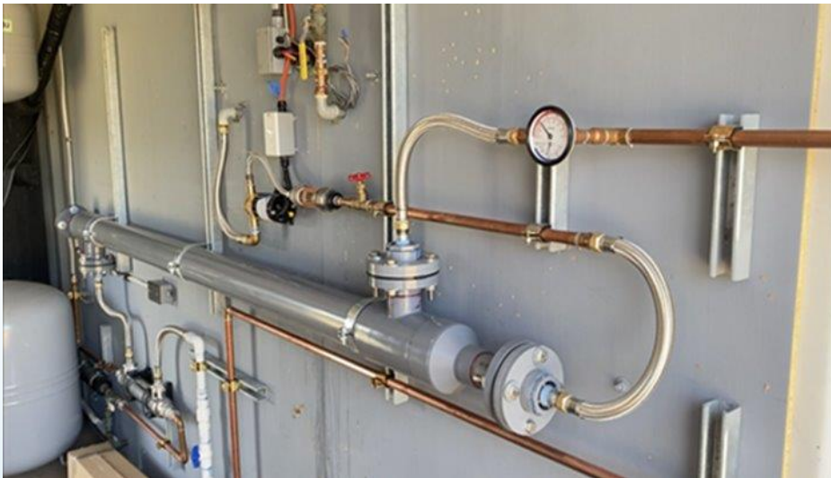
Wall-mounted plastic heat exchanger. Source: Trevi, Inc.
