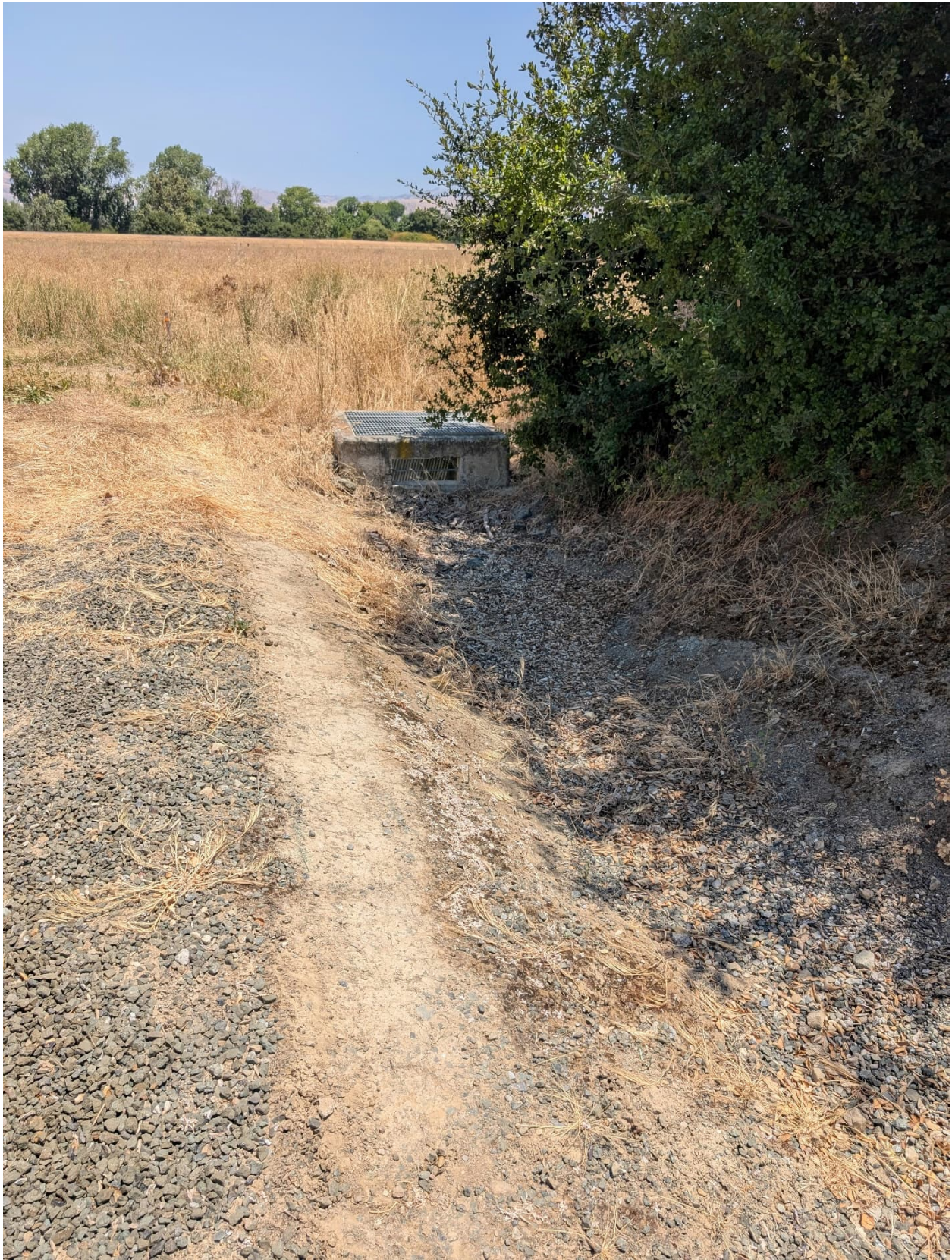
Photo 7. Ditch D-3 as viewed from the gen-tie alignment looking east. Drains to storm water capture system in the Los Esteros Critical Energy Facility. Photo taken on July 3, 2024.
