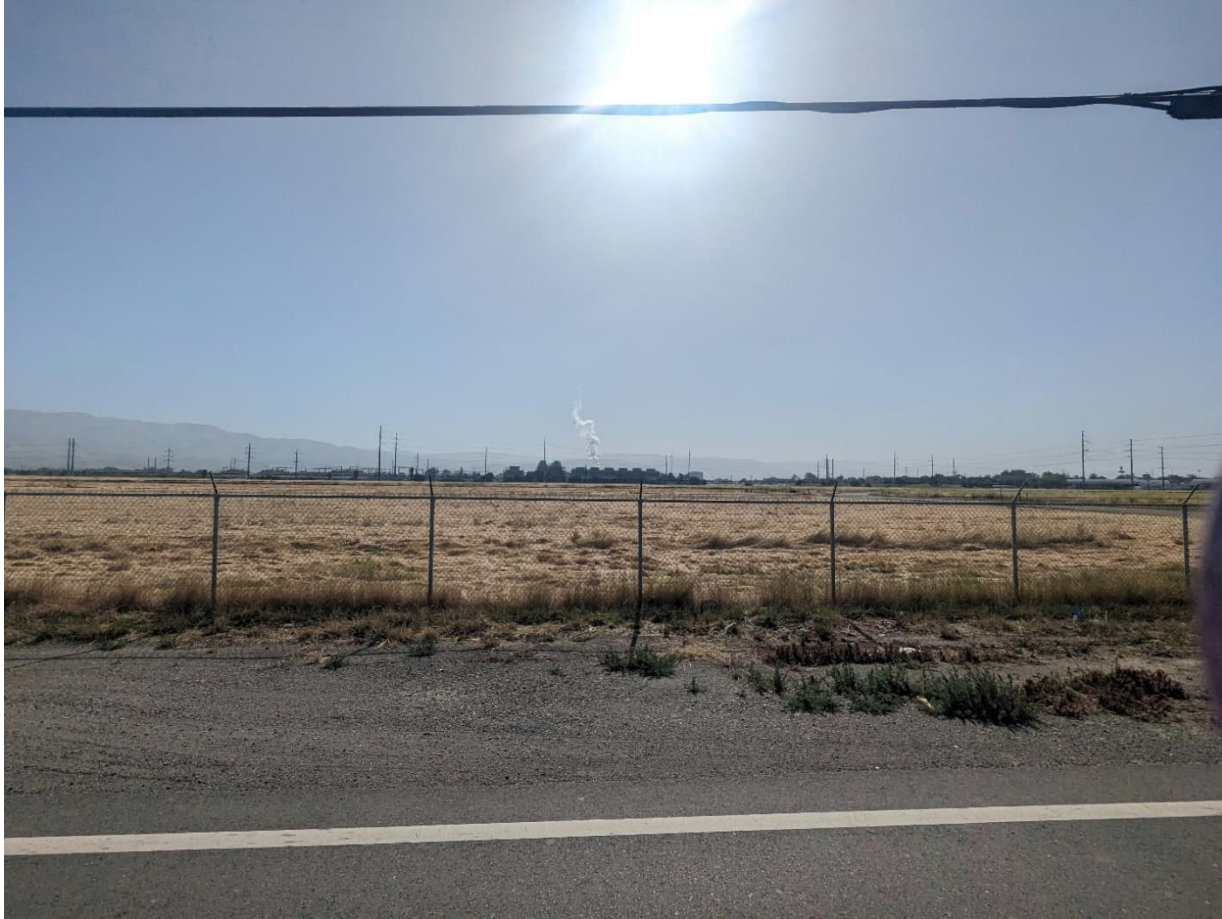
Figure 3. Looking East from Zanker Road toward the LECEF (Center) and Los Esteros Substation (Left)
