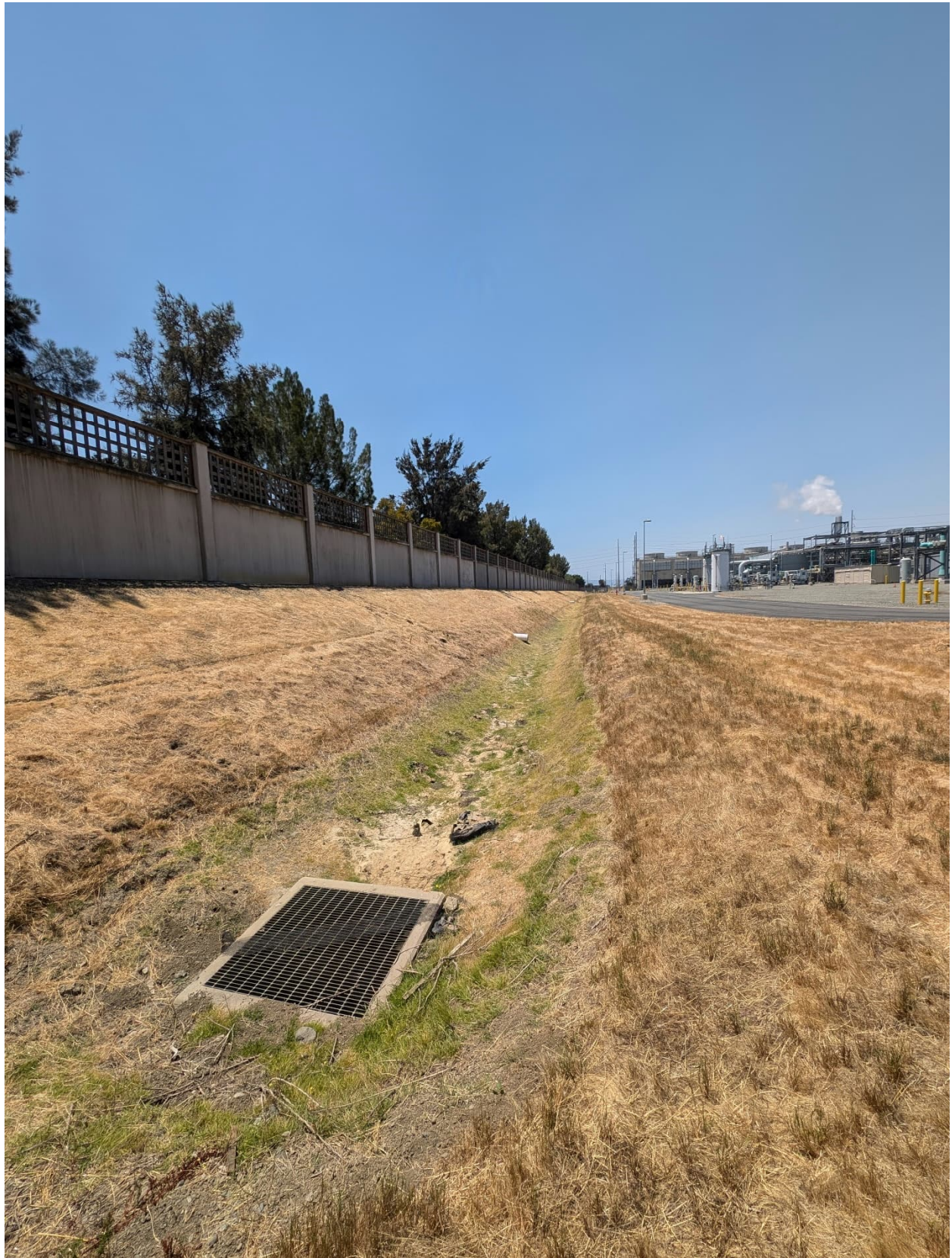
Photo 5. Ditch D-1 as viewed looking west from its eastern end. Drain leads to storm water capture system in the Los Esteros Critical Energy Facility. Photo taken on July 3, 2024.
