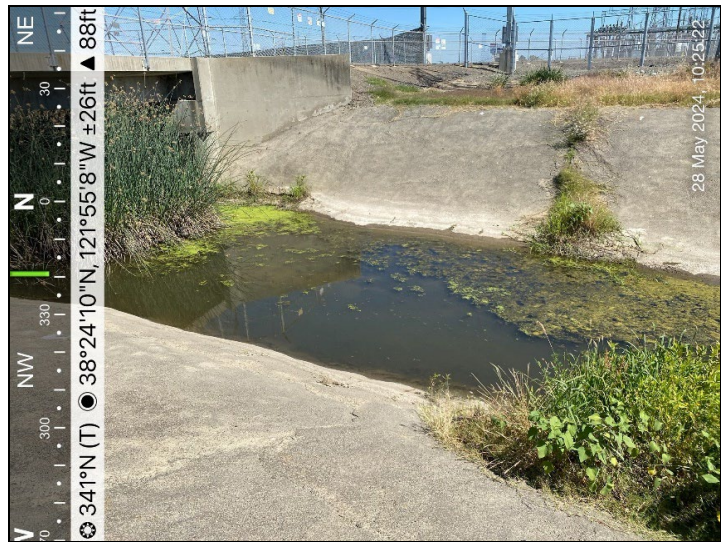
Figure 5. View Toward the Existing Vaca-Dixon Substation (view north-northwest; May 28, 2024).
