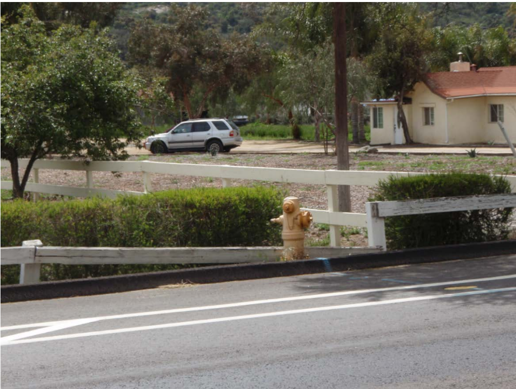
Fire Hydrant Along Valley Center Road
