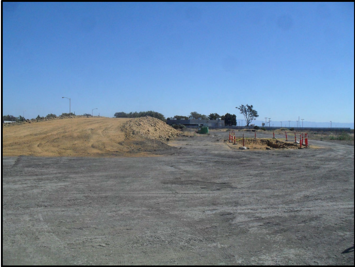
Laydown Area 5 – former metal fabrication facility
