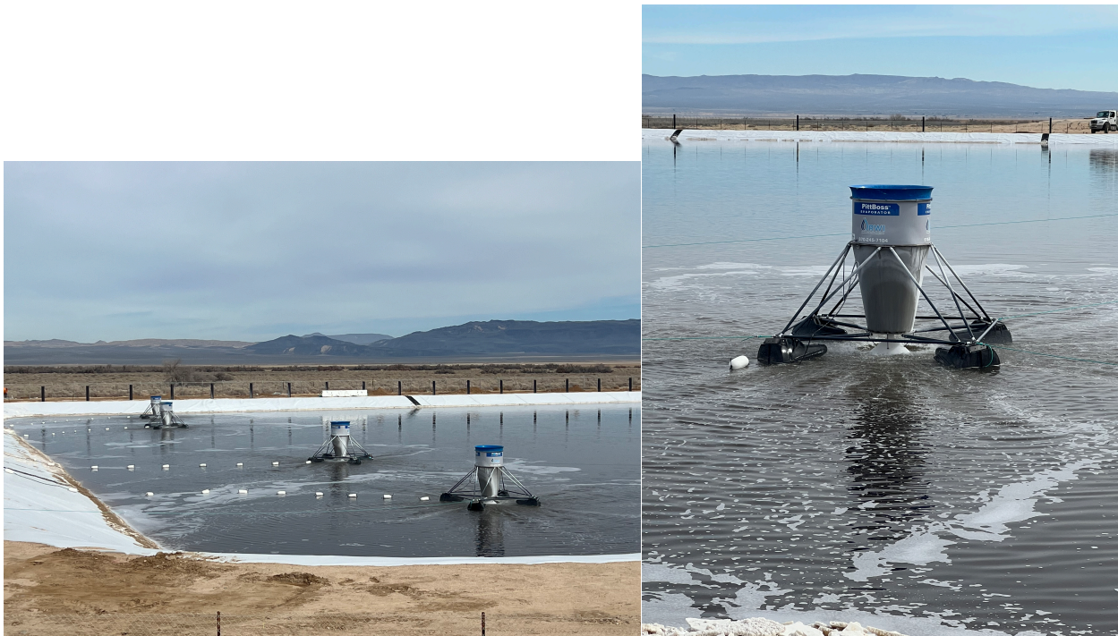
Photos 3&4: Location and close-up of PittBoss Sprayer-less Evaporators installed in the Alpha East Pond.
