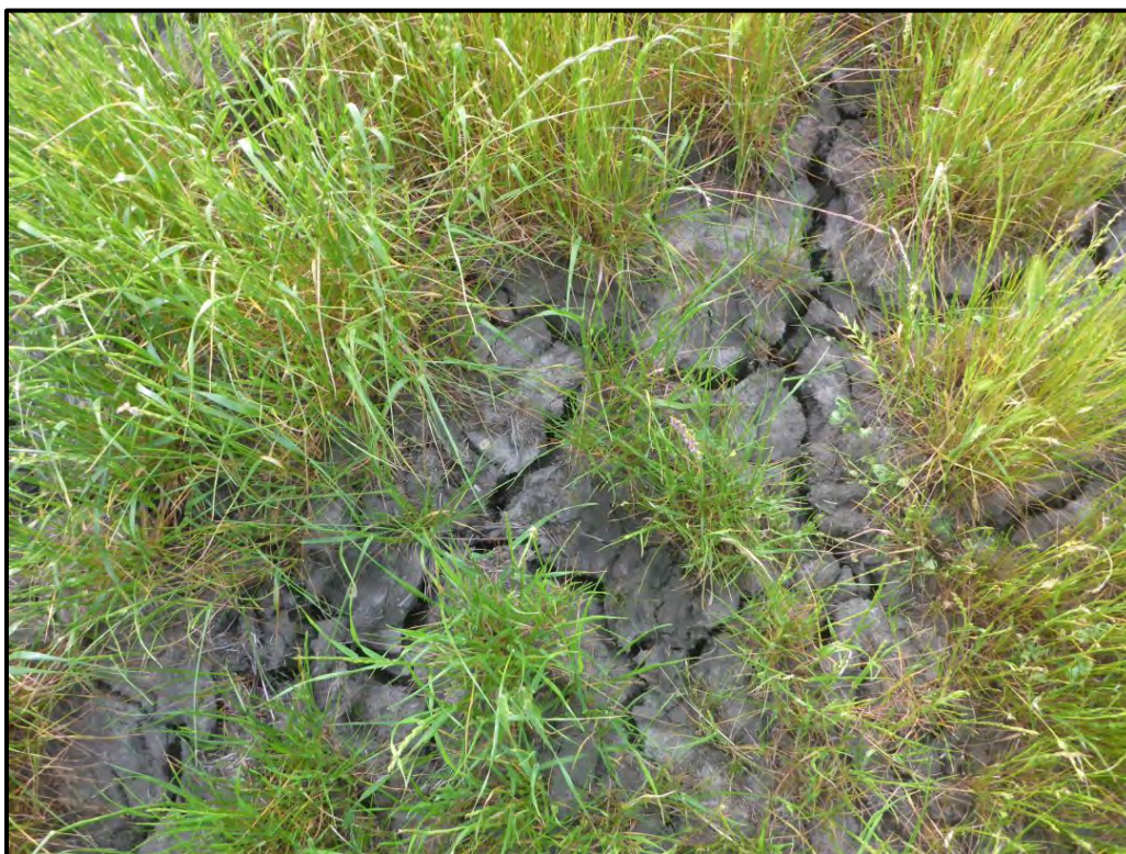
Photo 14. Cracking within clay soils, 2019.
