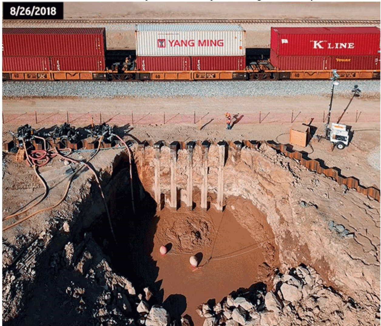
View of geoengineering attempts on moving Niland mud pot, next to Union Pacific Railroad line, from Lynch and Deane (2019).
