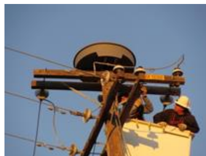
Installation of Osprey Nesting Platform
