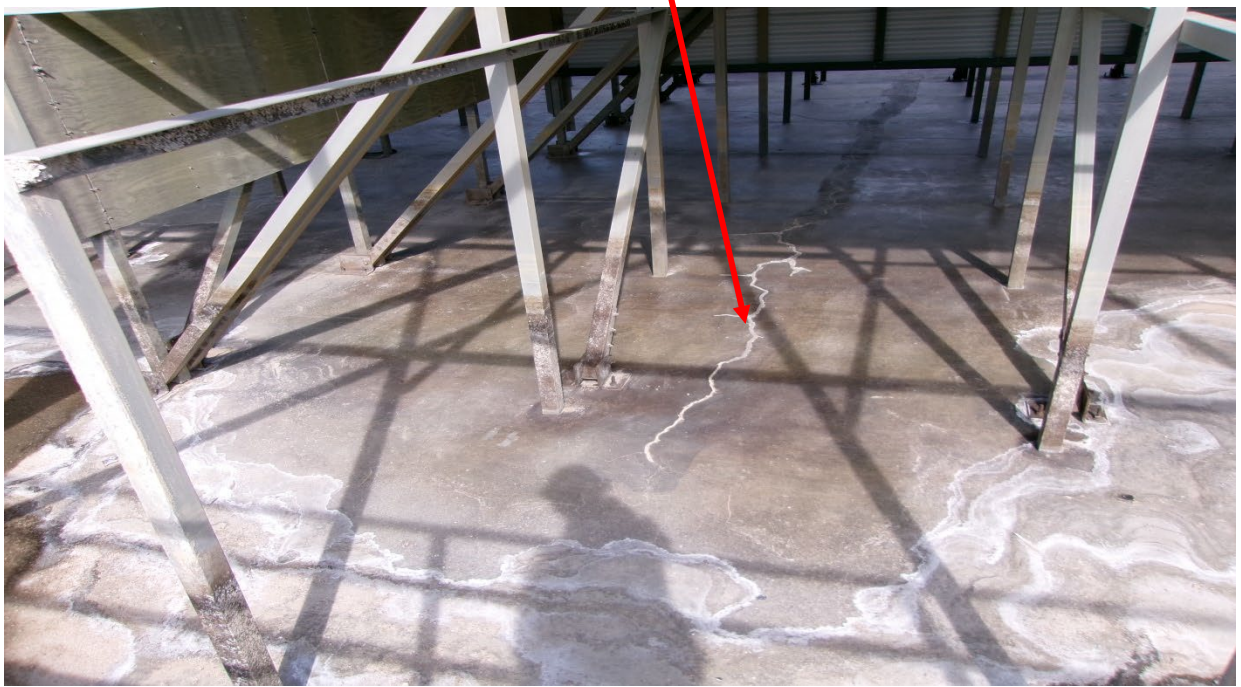
Cold Water Basin concrete cracks at random
