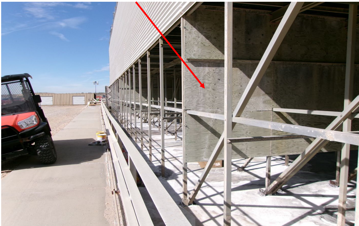
Fire wall partition walls by air inlet area good conditions
