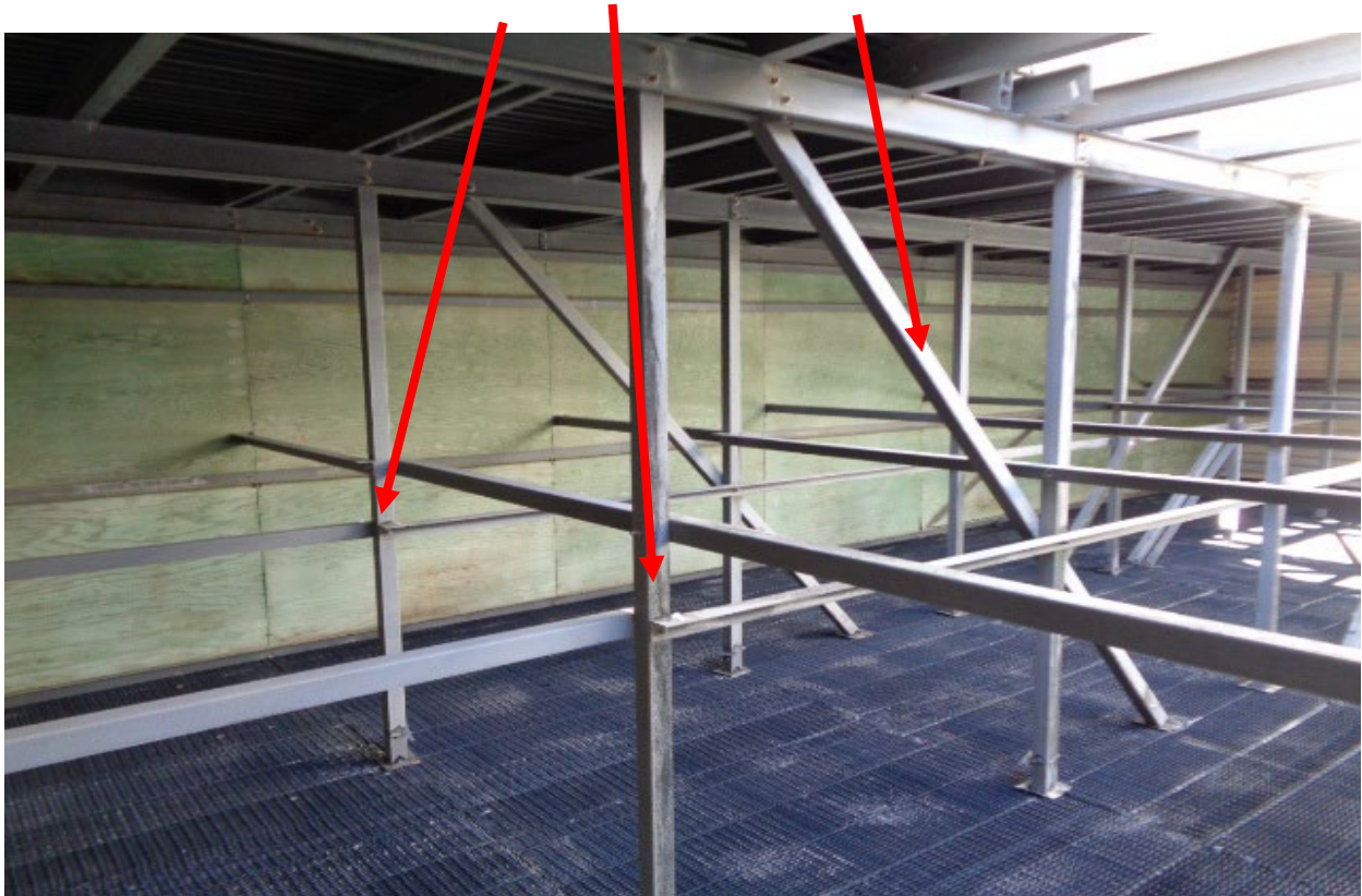
Air inlet Fiber Glass structure post, tie Lines, fill joist and braces good conditions
