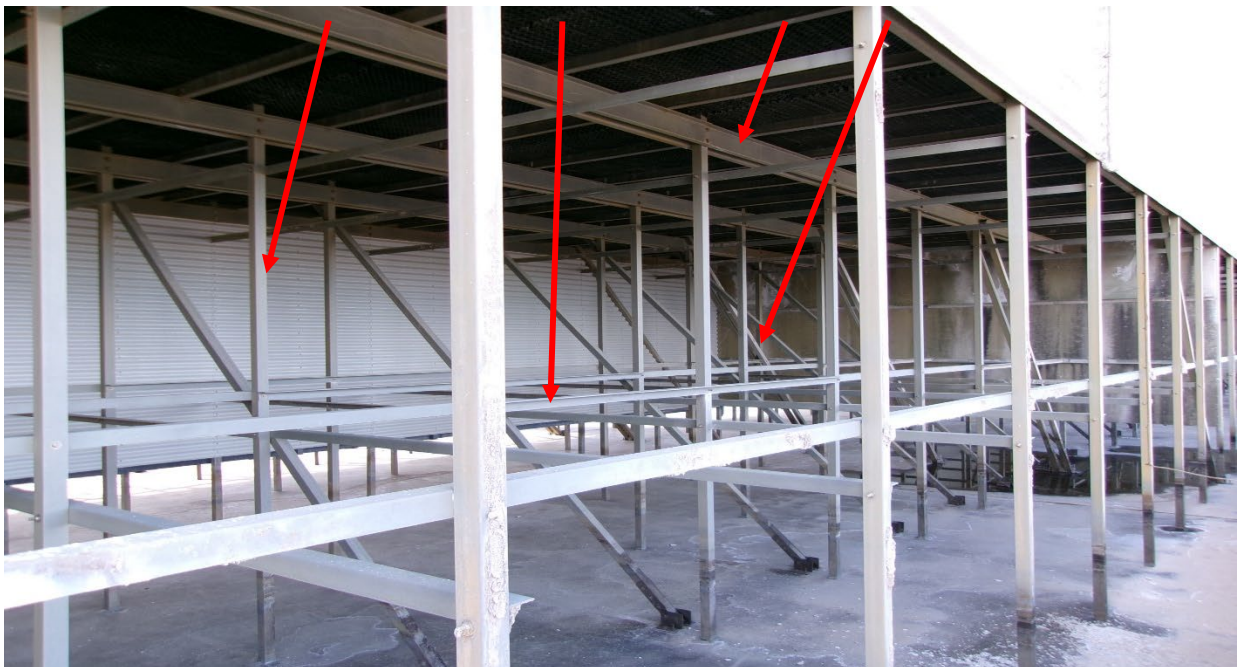
Air inlet Fiber Glass structure post, tie Lines, fill joist and braces good conditions
