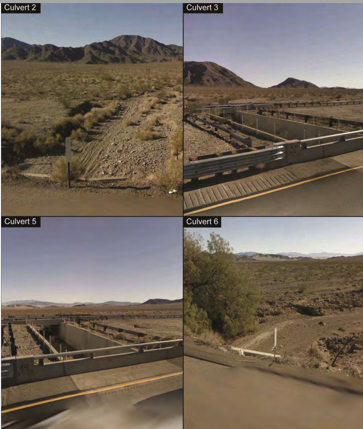
Figure 8: Box Culverts 2, 3, 5, and 6
