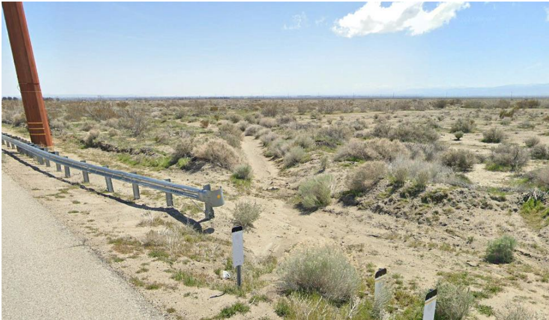
Photo 11. Looking southeast at the downstream portion of Drainage F on the south side of Rosamond Boulevard.
