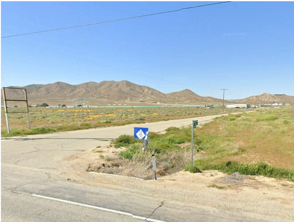
Photo 18. Looking northwest at Drainage J from the south side of Rosamond Boulevard.
