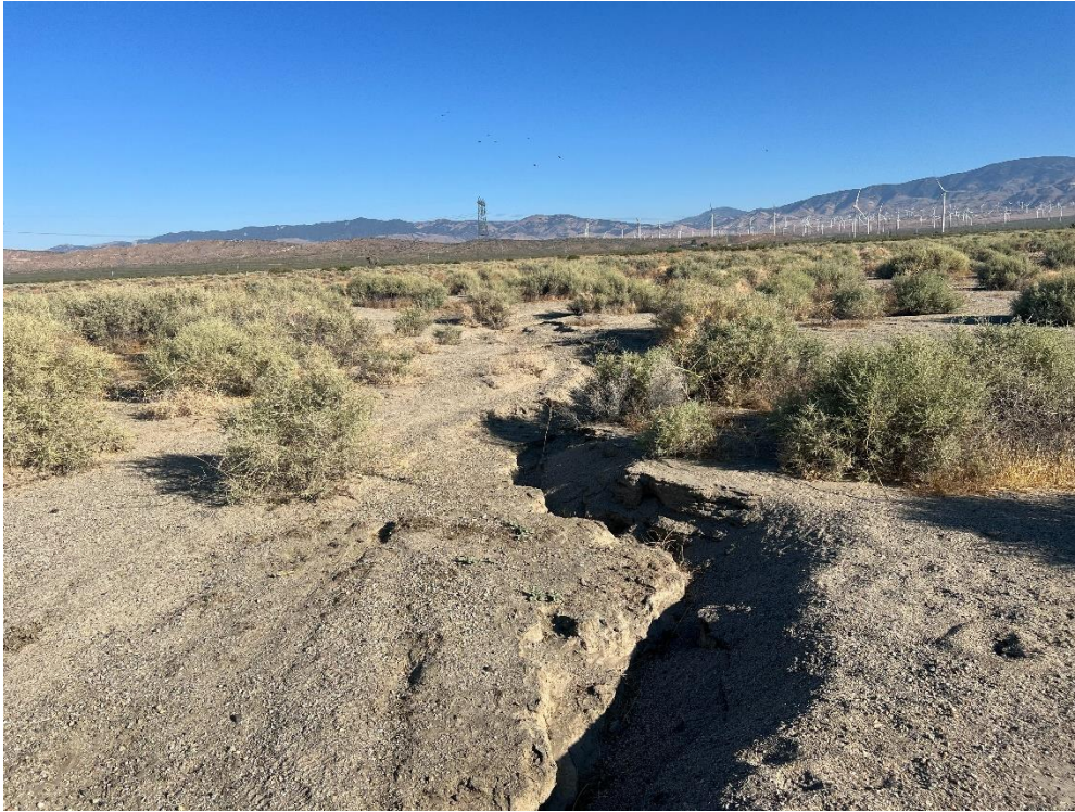
Photo 1. Looking north at Drainage A from the north side of Rosamond Boulevard.
