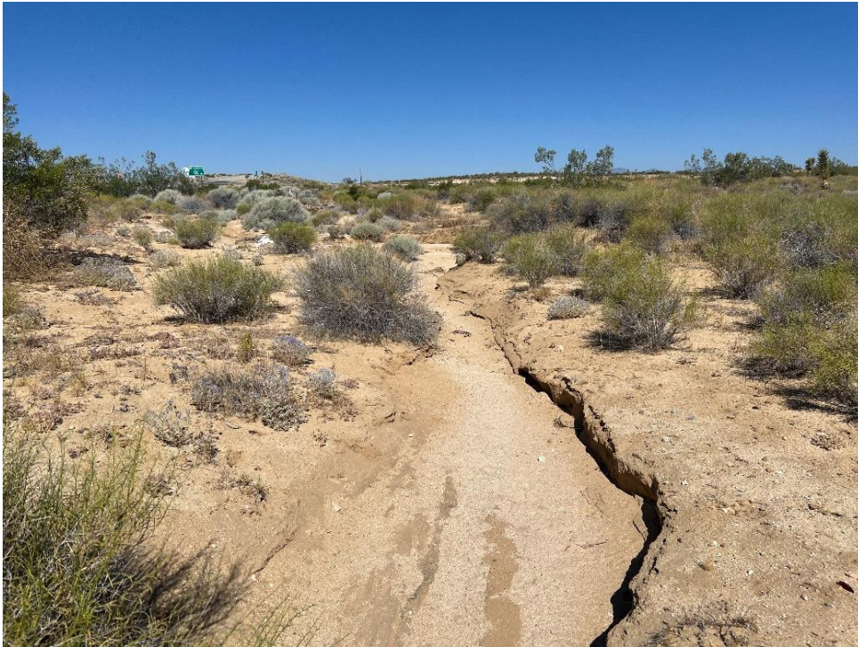
Photo 30. Looking west at the upstream portion of Drainage R from the north side of Dawn Road.
