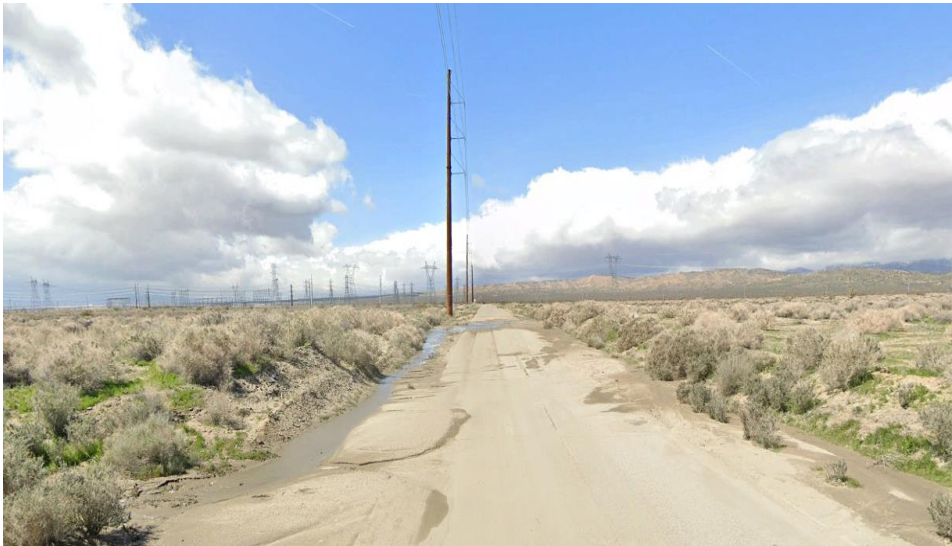
Photo 7. Looking west at the same area described in Photo 3. Photo was taken following a rain event to show run-off flowing down Rosamond Boulevard from Drainage A to Drainage B, the result of clearing sediment from the road and redirecting flows.
