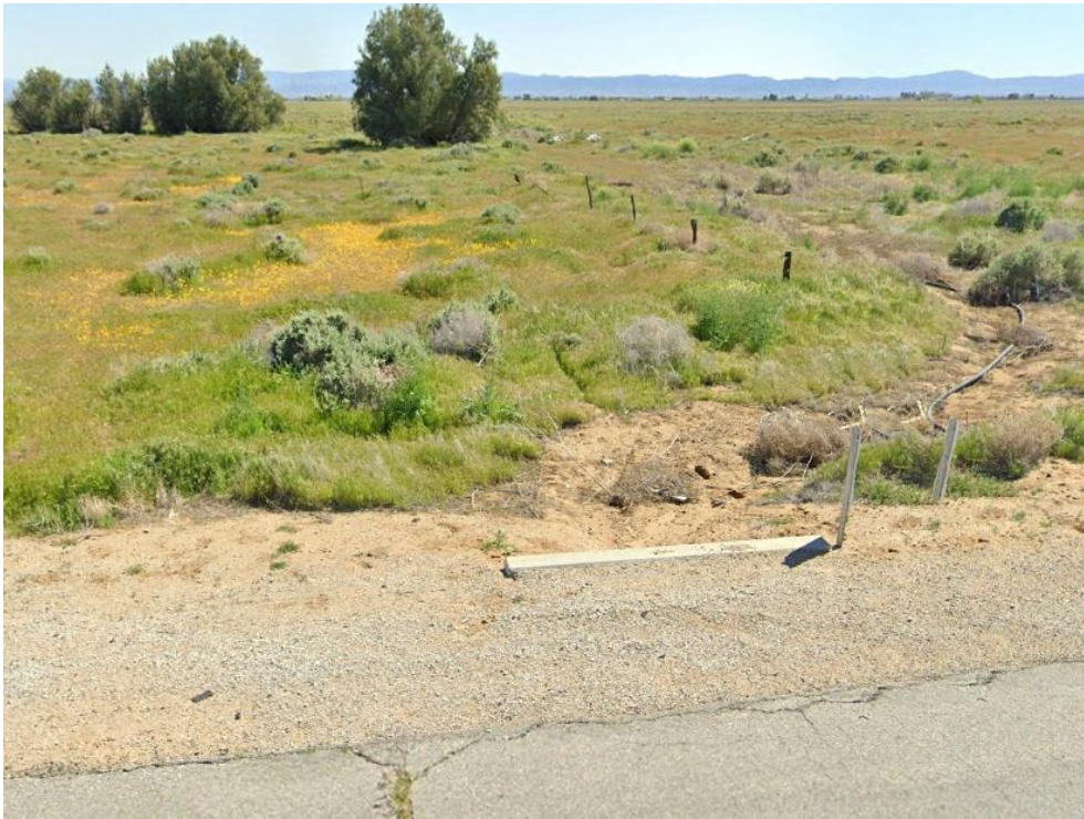
Photo 17. Looking south at the downstream portion of Drainage I on the south side of Rosamond Boulevard.
