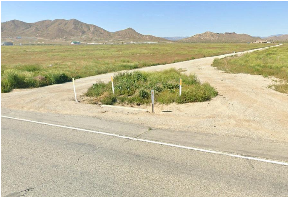
Photo 20. Looking northwest at upstream portion of Drainage K from the south side of Rosamond Boulevard.
