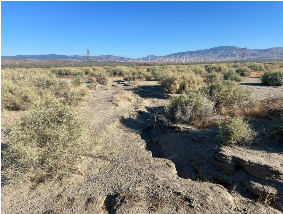
Photo 3. Looking north at the upstream portion of Drainage B on the north side of Rosamond Boulevard, at the end of the 200-foot buffer.
