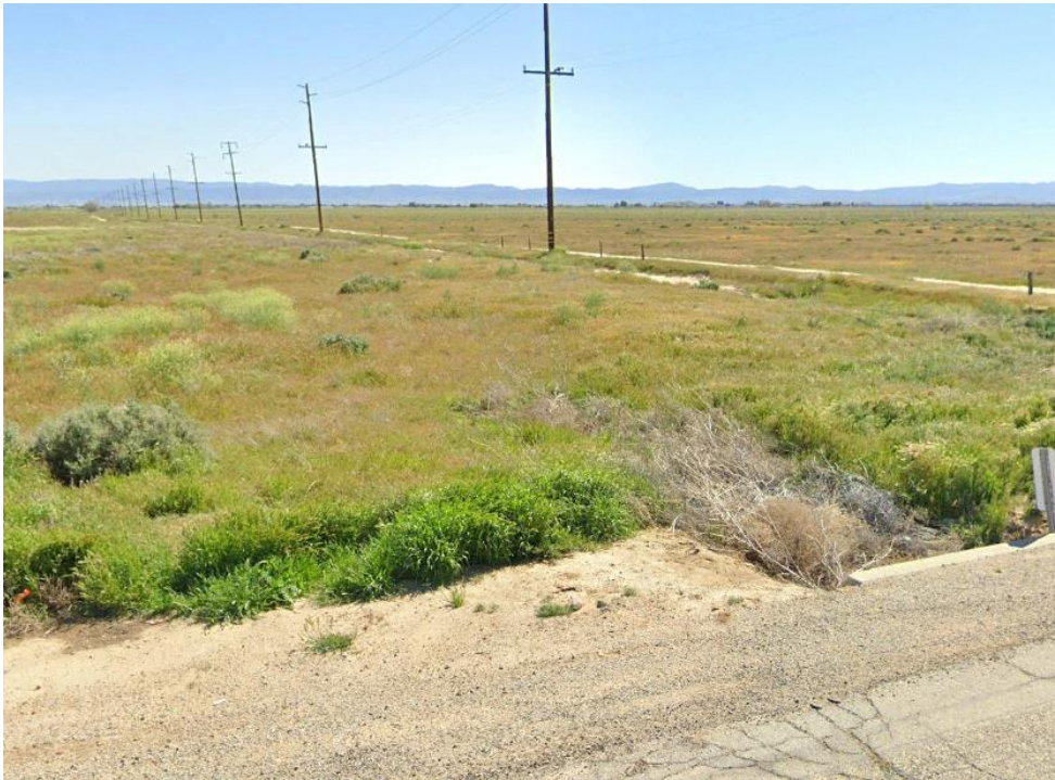
Photo 21. Looking southwest at the downstream portion of Drainage K on the south side of Rosamond Boulevard.
