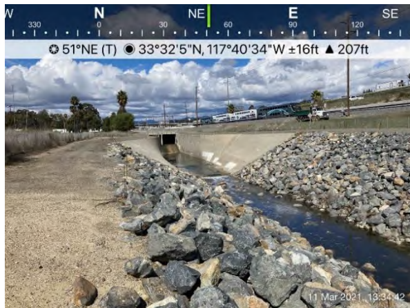
Photo 1: View of Oso Creek flowing out of culvert into non-vegetated channel at northeast corner of site.
