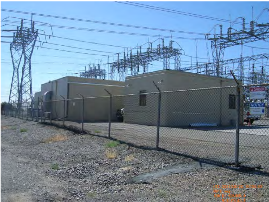
Photograph 3. Buildings No. 2 and 3, camera facing east
