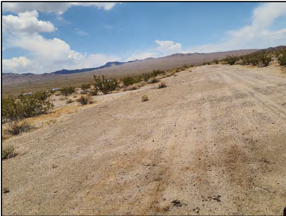
Photo C-10. SubArea A. 35.178669°, -116.166293°. Degraded paved dirt road lacking hydrologic indicators; indicators present outside road prism.
