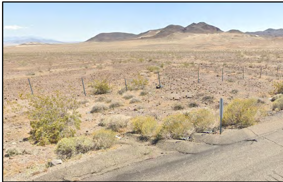
Figure 21. Example of a highway water chute/flume where there is a break in the asphalt highway berm; view from the highway, facing the project site.
