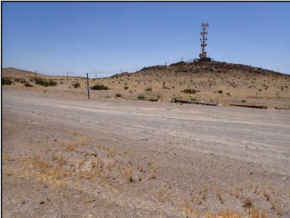
Photograph 8. Cell tower located southwest of the subject property.
