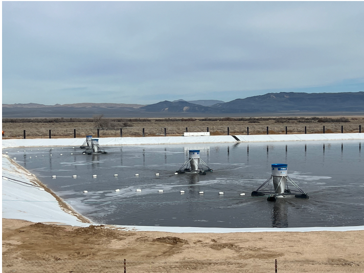
Photos 3&4: Location and close-up of PittBoss Sprayer-less Evaporators installed in the Alpha East Pond.
