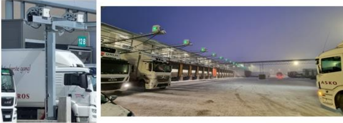
Figure 2. Charging Site with Overhead Charging Dispensers
