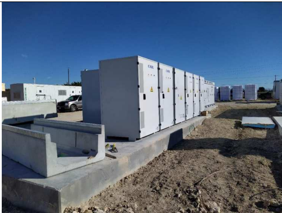
Photo 4 – BESS modules placed on concrete foundations during construction.
