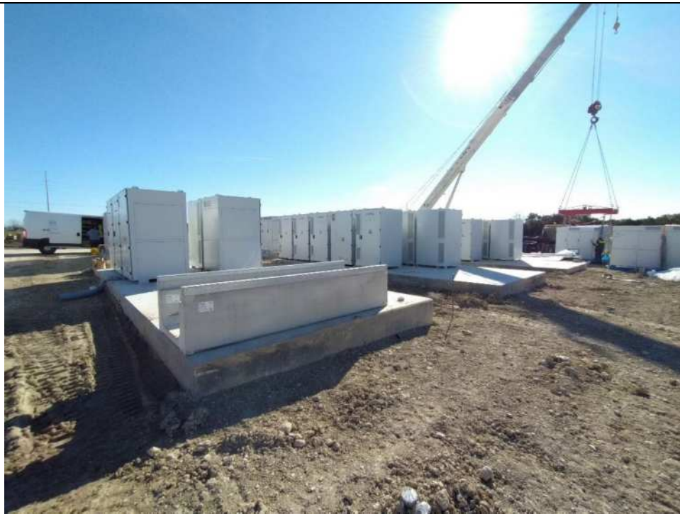
Photo 1 – BESS containers being placed on concrete pad sites during construction.
