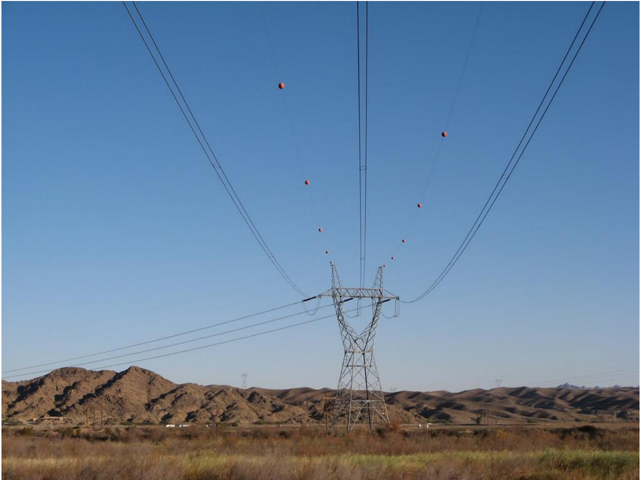
The 500kV Southwest Powerlink transmission line, as seen from Imperial County Route 24
