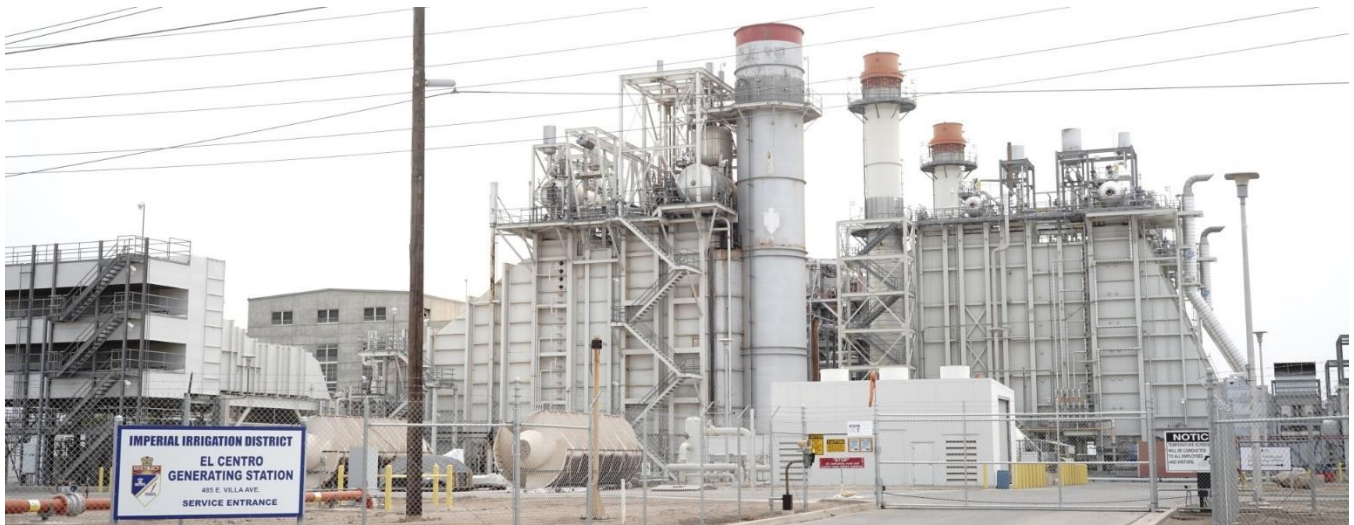
El Centro Generating Station in El Centro, California.
