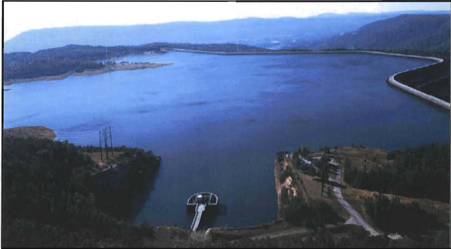
Man-Made Upper Reservoir of TVA's Raccoon Mountain PH Plant Operational Date: 1979; Capacity: 1620 MW; Max. Discharge Duration: 22 hrs
