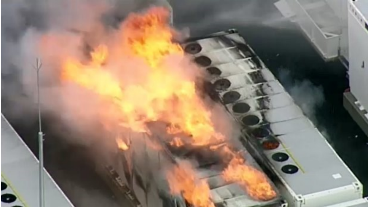
Figure 3. Containerized BESS After Thermal Runaway Initiates.
