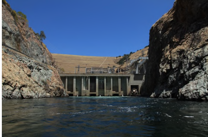
Figure 16. Don Pedro Hydroelectric Power Plant
