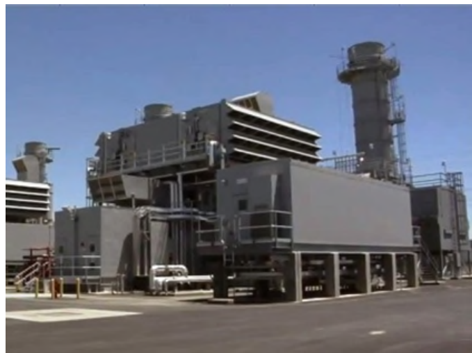
Figure 10. Almond II Power Plant
