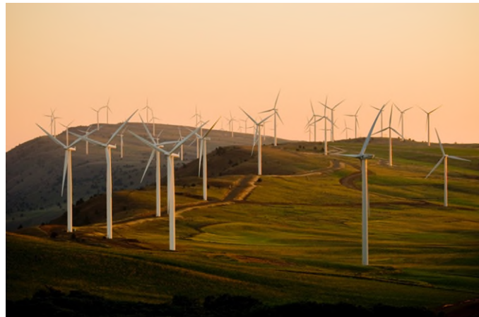
Figure 14. Tuolumne Wind Project Power Plant
