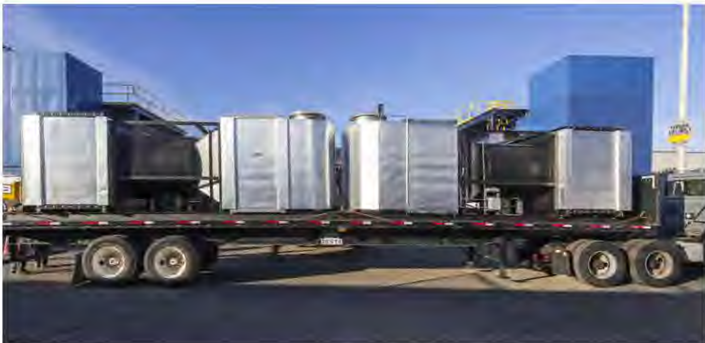
Two factory assembled CompactSCRT systems arriving at the jobsite. A single crane lift per unit eases installation.
