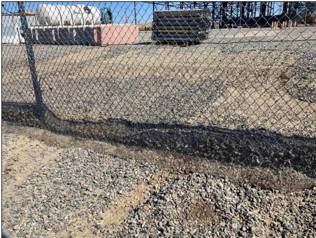
**Photo 34. Portion of the southwest fence showing signs of erosion. Holes in the fence were filled in by CGS Compliance Manager and BM on July 12<sup>th</sup>, 2023.**
