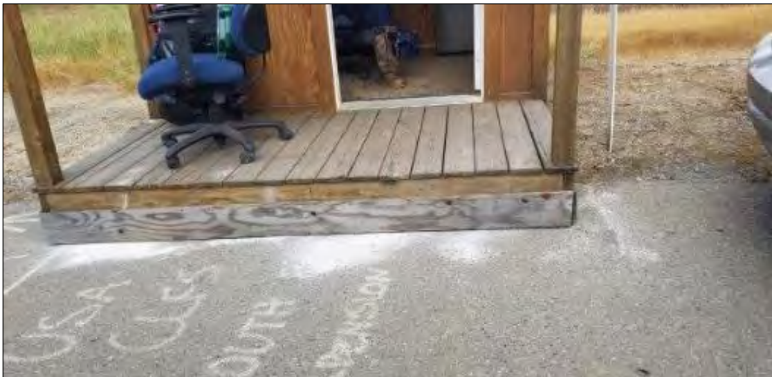
Photo 6. Snake board installed on guard shack on March 17 th , 2022.
