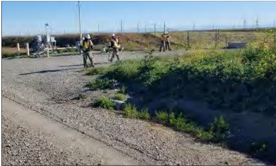
Photo 10. Weedeating at the Tehama Colusa canal on March 22 nd , 2022.
