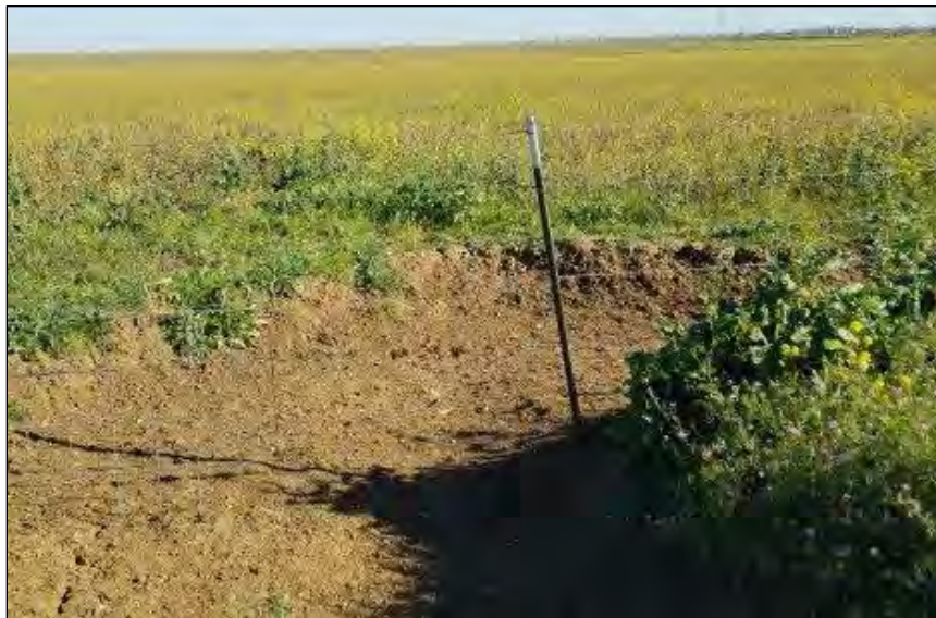
Photo 13. Hole near perimeter fence in the northeast corner of the site on March 23 rd , 2022.
