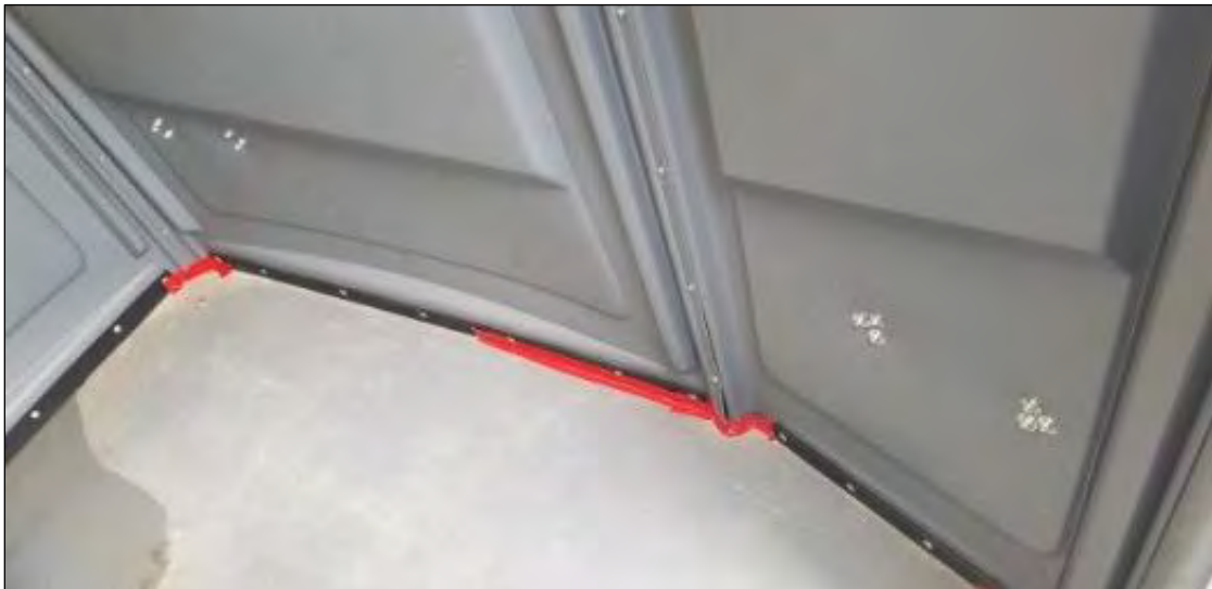
Photo 7. Holes in guard shack porta-potty taped off to exclude wildlife on March 17 th , 2022.
