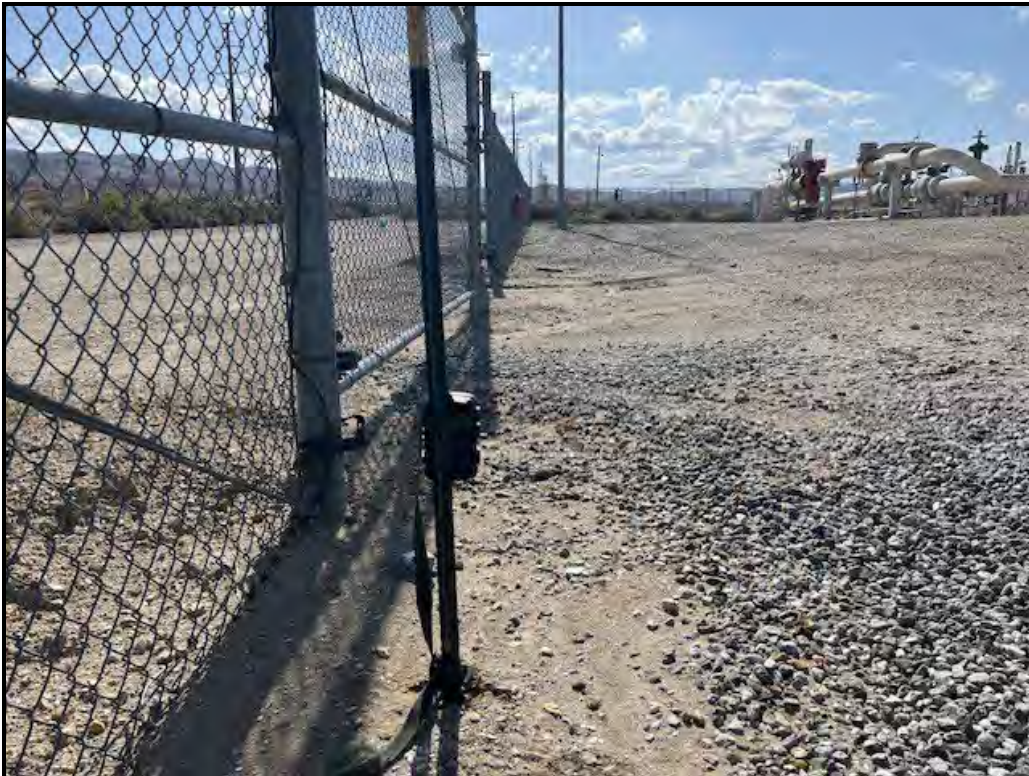
CT03 (35.20963, -119.58579): Located inside the perimeter fencing at a gap beneath a gate in the southwestern portion of the Site
