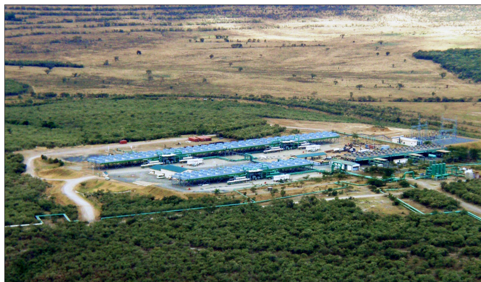
Figure 2. Olkaria III binary plant with air cooled condensers (Ormat).
