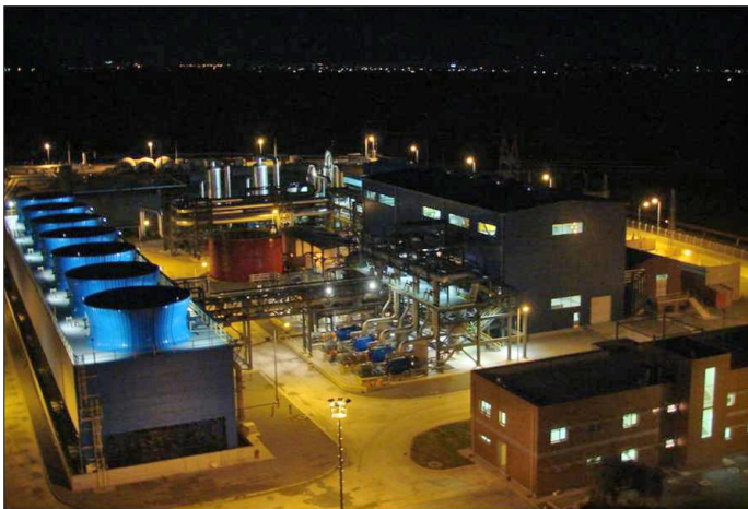
Figure 1. Germencik flash plant with wet cooling tower.
