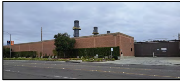
Miraloma Avenue, south wall (1/24/24)
