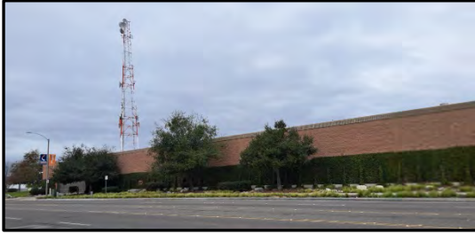
Miraloma Avenue, south wall (1/24/24)
