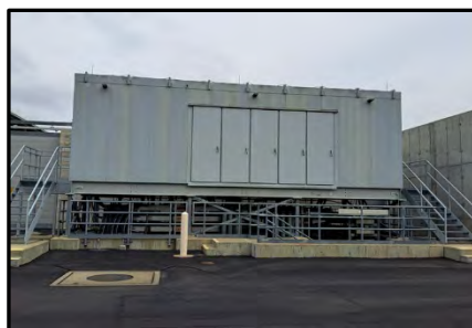
Balance of Plant Building (1/24/24)
