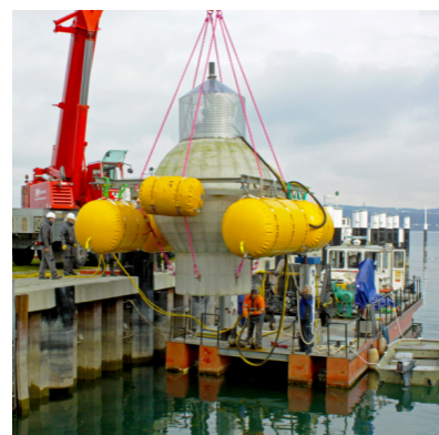
Fig. 2: Photos of the fabrication and 1/10 scale testing of Fraunhofer's first-generation subsea pumped hydroelectric system, StEnSEA.
