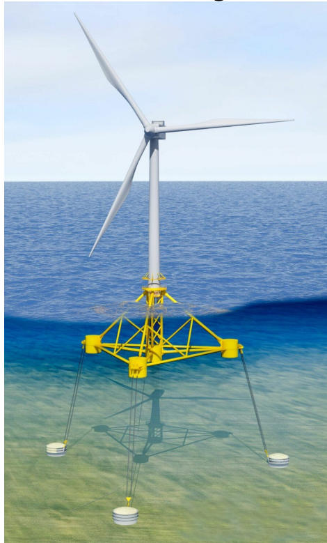
Figure A-5: SBM Tension Leg Platform Concept
