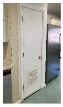
Figure 22: DHW closet door with lower grilles from a small commercial kitchen in Woodland, CA.
