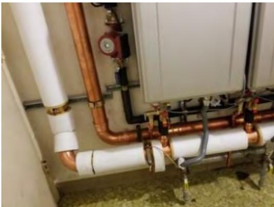
**Figure 2: Field observation punch list photo showing missing pipe insulation.**
