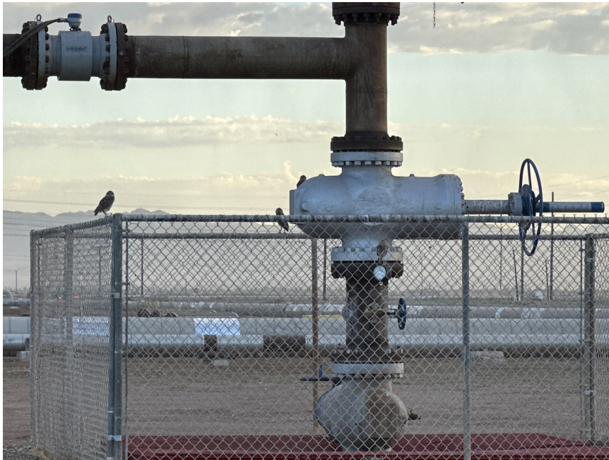
Photograph 24: BUOW_60 – Burrow near injection well head in ENGP BSA. This well is not managed by the IID.
