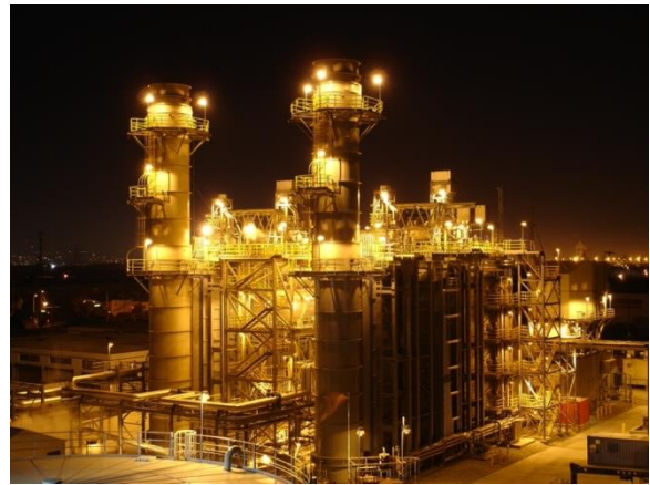
Figure 47. Malburg Generating Station
