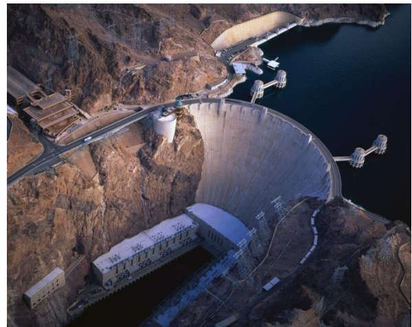
Figure 50. Hoover Dam Hydroelectric Power Plant
