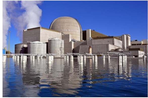
Figure 49. Palo Verde Nuclear Station
