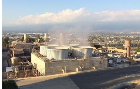
Figure 51. Puente Hills Landfill Gas Plant
