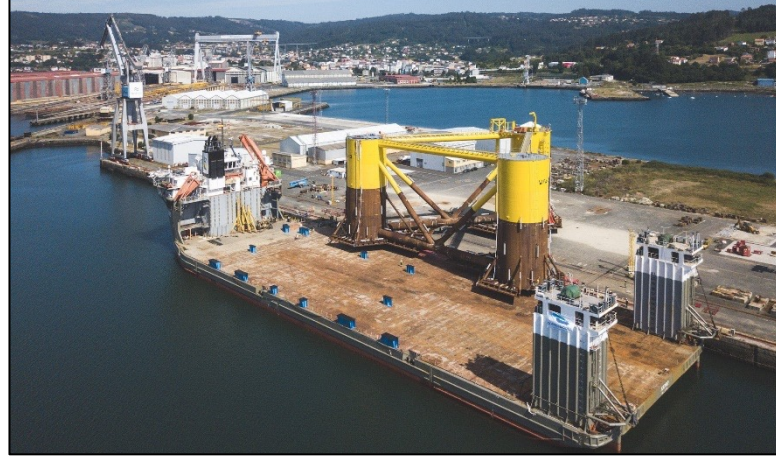
2) Loadout onto semi sub
