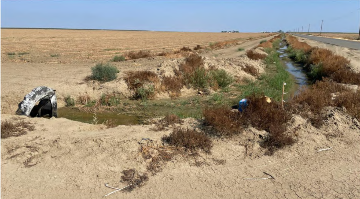
Photograph 14. View north, AD-6, Photo Point 11. View at the intersection of West Harlan Avenue and South Sonoma Avenue. AD-6 has an average width of 5 feet and is connected to AD-5 through the culvert seen on the left. This section is also generally trapezoidal in shape, and a slope break can be seen on the bank near the center of the photo. Vegetation is Russian thistle and bearded sprangletop. AD-6 continues north along South Sonoma Avenue, within the 250 foot buffer of the Project site. AD-6 flows through a culvert into canal AC-1 approximately 0.5 miles north. AC-1 averages 40 feet in width and is connected on the north to AC-2, averaging 65 feet in width, which runs offsite. While supporting vegetation occasionally, these ditches and canals are maintained regularly and generally kept free of vegetation. An OHWM data sheet was prepared for this feature in the approximate location of the upper right of this photograph and is attached in Appendix J.
