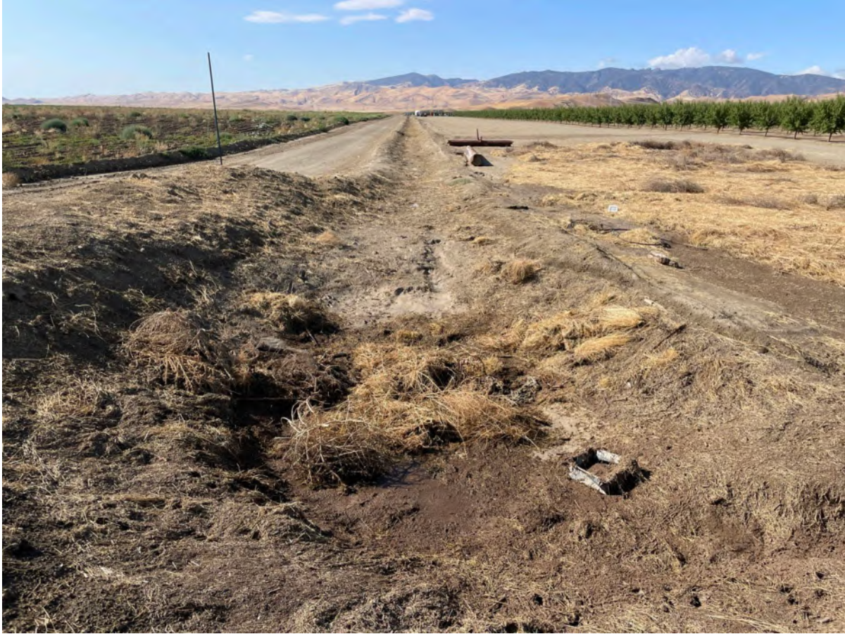
Photograph 9. View south, AD-1, Photo Point 1. Typical of larger, primarily u-shape agricultural ditches with natural line on bank and slight erosion creating slope break where water enters the ditch. Average OHWM width is 8 feet. Ditch is non-jurisdictional as it is for agricultural purposes. An OHWM data sheet was prepared for this feature in the approximate location of center of this photograph and is attached in Appendix J.
