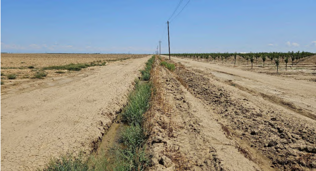
Photograph 11. View east, AD-5, Photo Point 9. AD-5 is typical of trapezoidal ditches throughout the Project site. The average OHWM width is 3 feet, often widening somewhat at culverted crossings. By design the ditch has a bed and banks, other indicators include break in slope and natural line on bank. In some reaches the ditch is vegetated, here with Russian thistle and further west includes bearded sprangletop ( Leptochloa fusca subsp. fascicularis ) (NL) and other non-hydrophytic vegetation. This ditch was being actively maintained during the survey by a crew removing vegetation further to the east.
