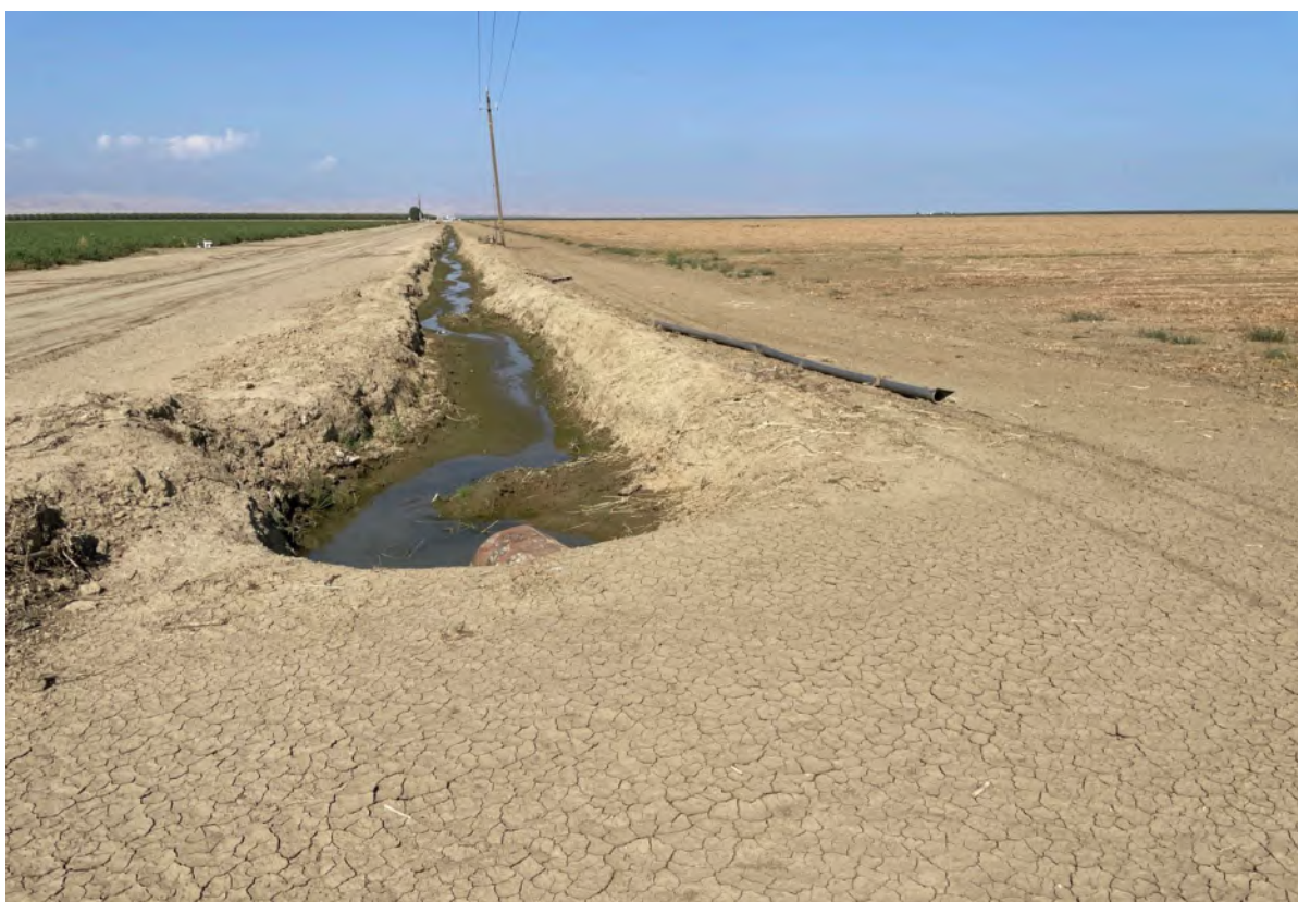
Photograph 13. View west, AD-5, Photo Point 12. View of typical culvert crossing of ditch AD-5. Average size of culverts is 30-inches.
