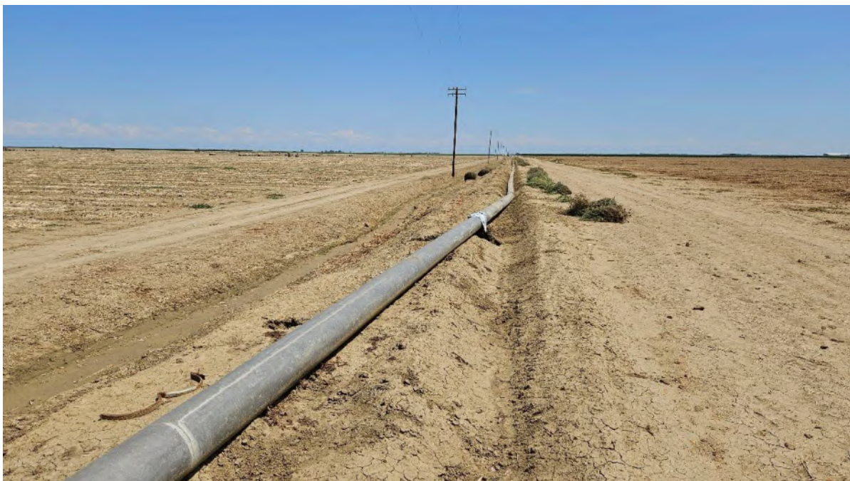
Photograph 12. View east, AD-5, Photo Point 10. AD-5 is on the left in the photo, parallel on the right is a pipe v-ditch with Russian thistle that has been removed to lay the pipe.
