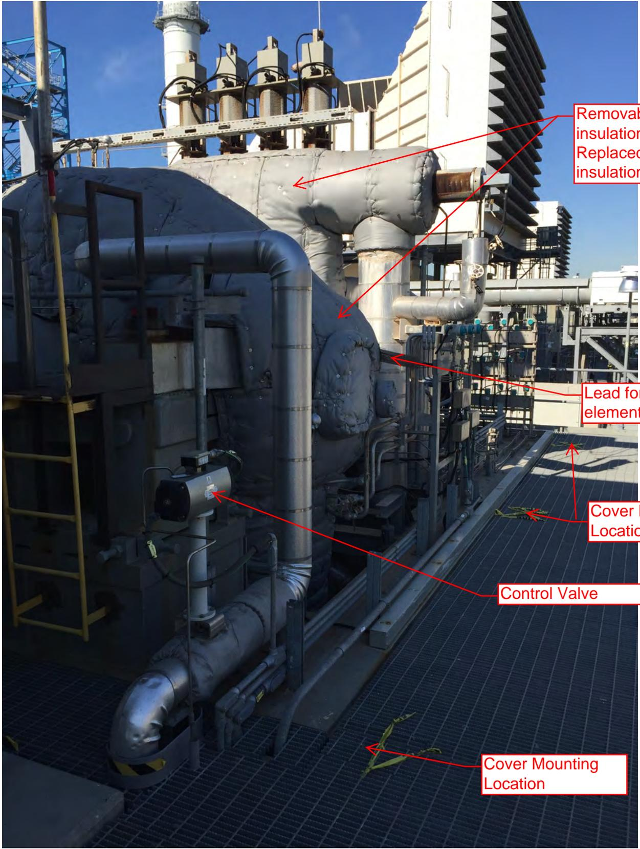
Removable insulation pads. Replaced plaster insulation.
