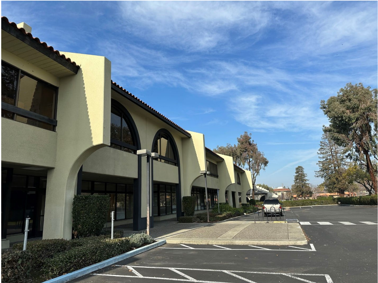
View of parking lot, existing building, and landscape area on the eastern side of the site. IMG_2532.JPEG, taken by Leane Dunn, December 23, 2022.
