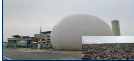
Biogas production plant
