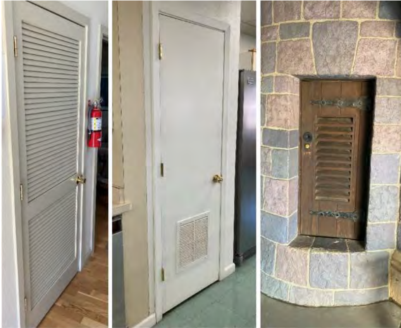
Figure 47: Examples of louvered closet doors and retrofit grilles installed.
