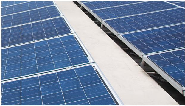
Mechanically attached racking systems can reduce maintenance costs. Photo courtesy of Fidelity Roof Company.
