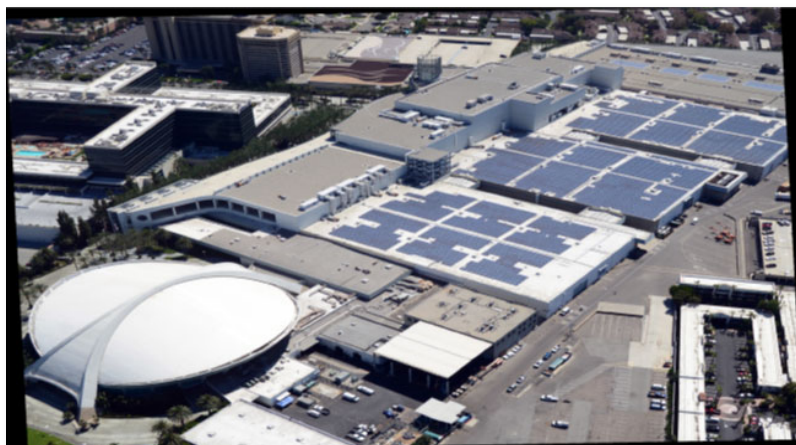
Photo 6: The 2.4 MW Anaheim Solar Energy Plant at Convention Center
