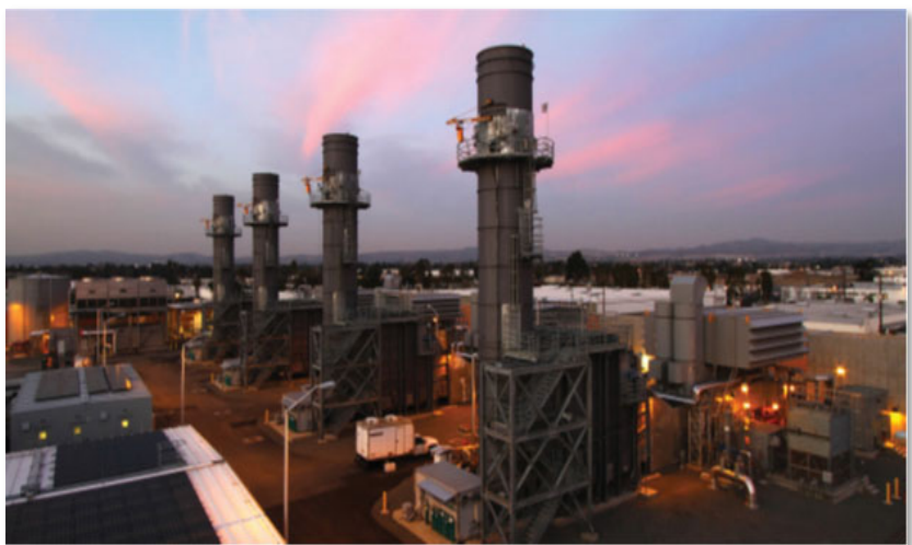
Photo 4: Canyon Power Plant
