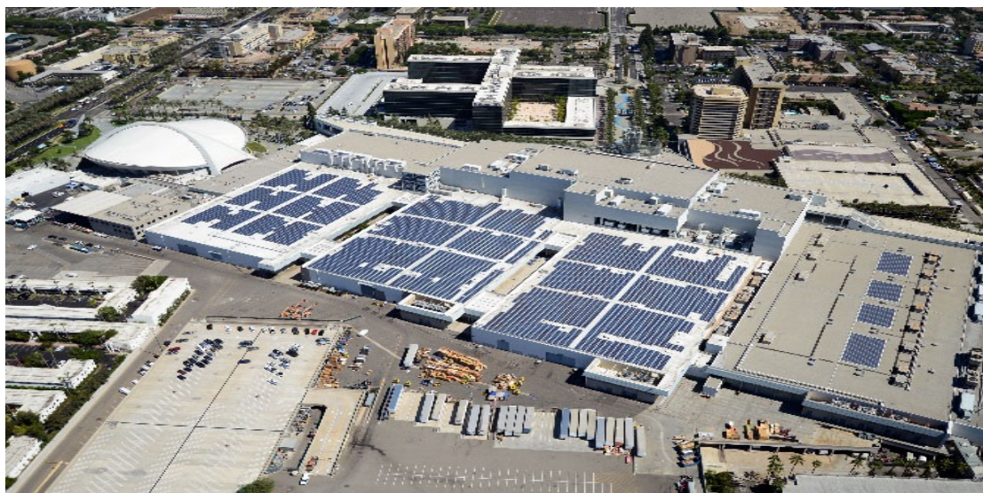
Photo 13: Solar PV System on the Roof of the Anaheim Convention Center
