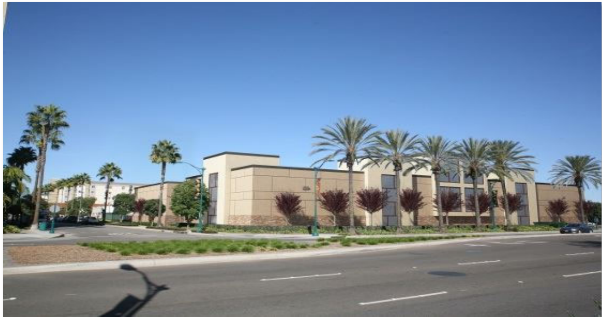
Photo 1: Harbor 69/12kV Substation
