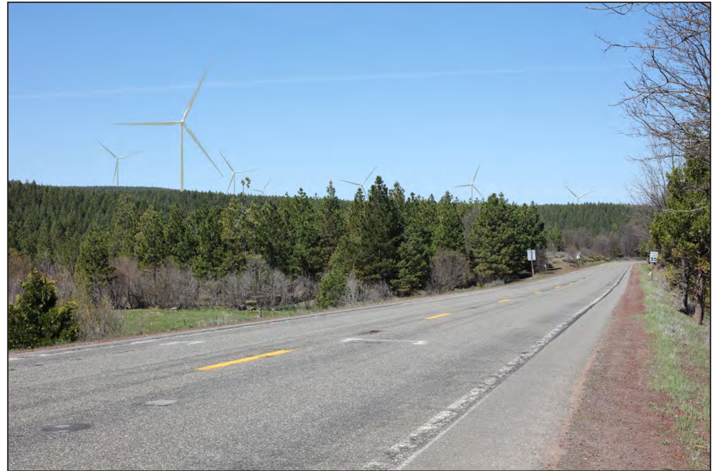
b) Simulated view from KOP 4a. Project turbines would be visible to different extents at distances of 0.8 mile to 3.4 miles away.
