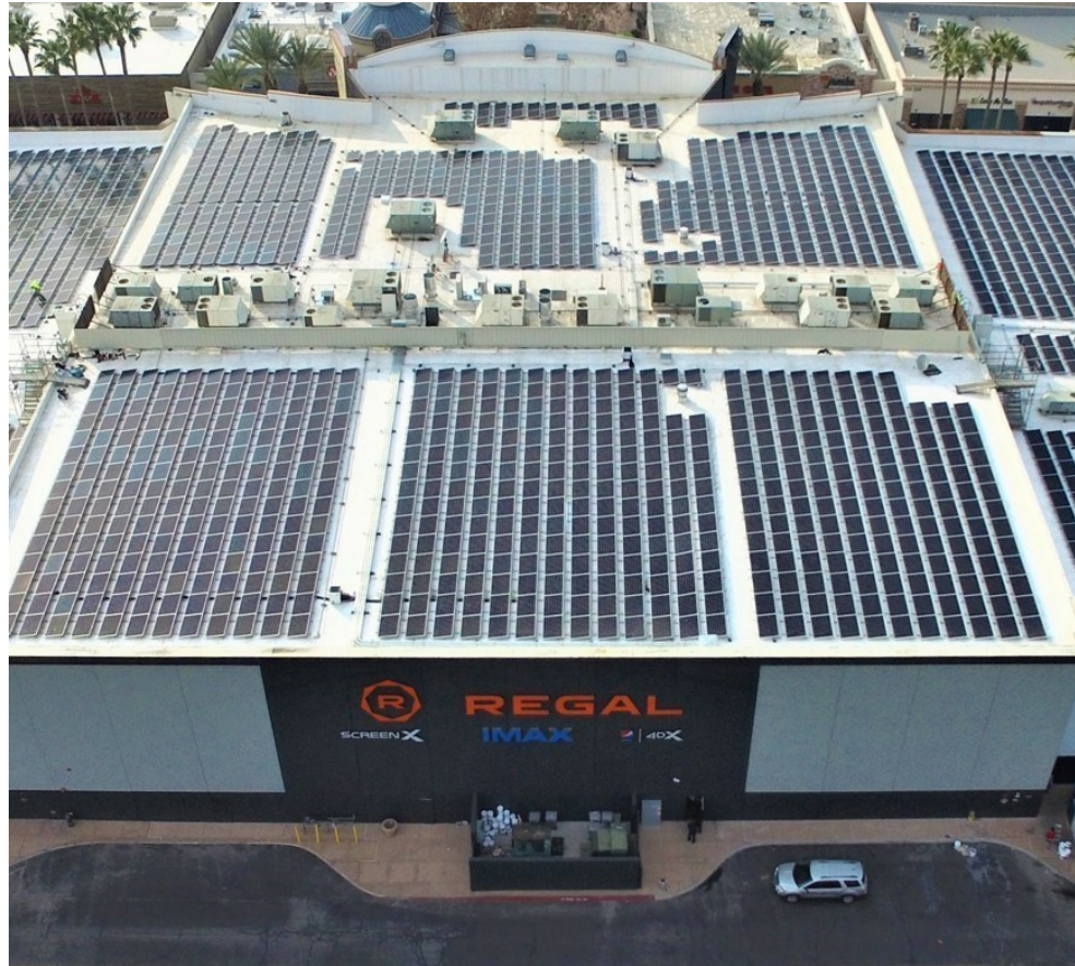
Regal Cinemas (Fresno, Ca) 756KW Ballasted Roof Mounted
